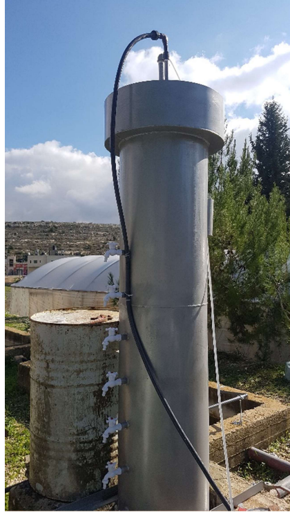
Photo 3.1: Constructed Pilot Scale UASB-septic tank installed at BZU Campus
