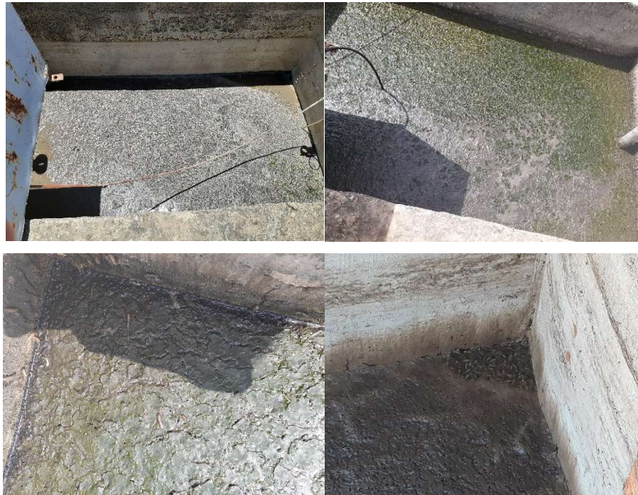
Photo 4.3: Feed storage tank prior mixer installation (August, 2019)
